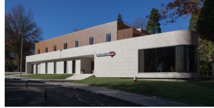
Ronald McDonald House in Porto Hospital de S. João, Porto, PT | 2010 - 2013
