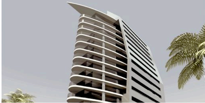
Multipurpose Building in Oran Djamel Mehiaoui Oran, Republic of Algeria, DZ | 2014
