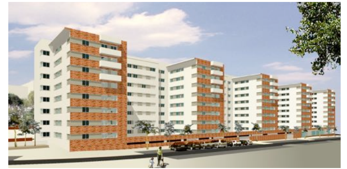
Low Cost Residential Buildings in Lisbon RQ2 Urbanização do Vale de Chelas II, Lisboa, PT | 2001 260 apartments
